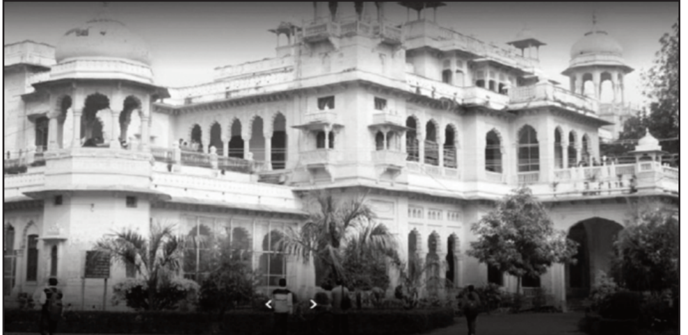
Allahabad University campus and Administrative Building
